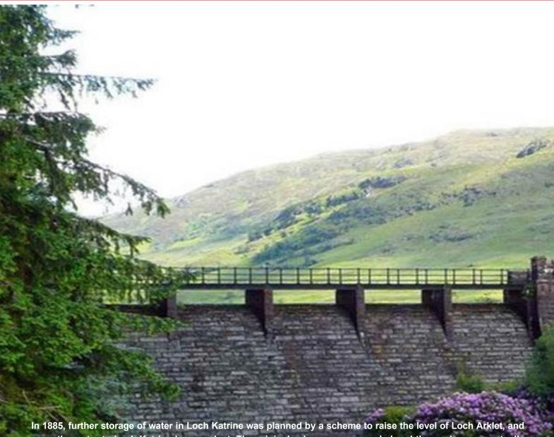
In 1885, further storage of water in Loch Katrine was planned by a scheme to raise the level of Loch Arklet, and carry the water to Loch Katrine by aqueduct. The original scheme was amended and the work was eventually carried out from 1909 - 14. The dam across Loch Arklet's outlet is 350 yards long and made of concrete faced with red freestone from Annan. It is 35ft high and 11ft wide at the top.
