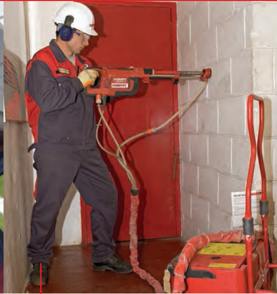
Slurry Containment and Re-cycling System
