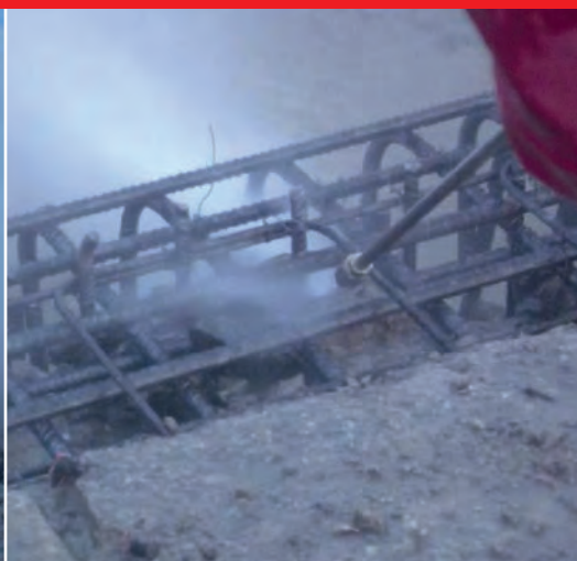
Preparation of Reinforcement prior to Reinstatement of Concrete
