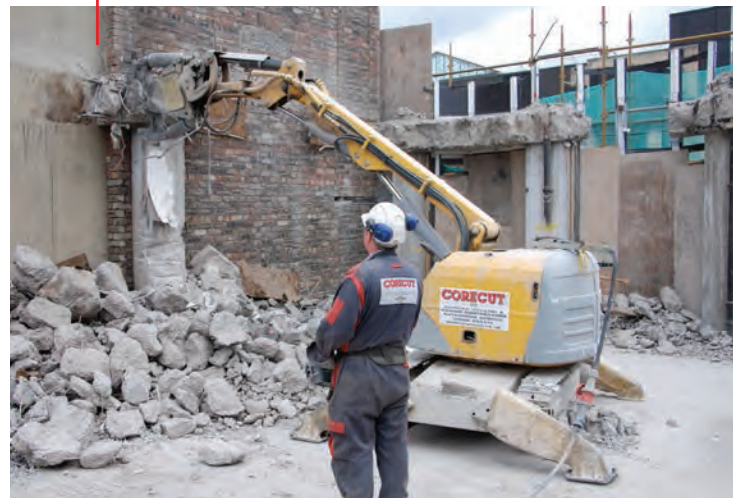
Remote demolition of 500 mm thick roof structure
