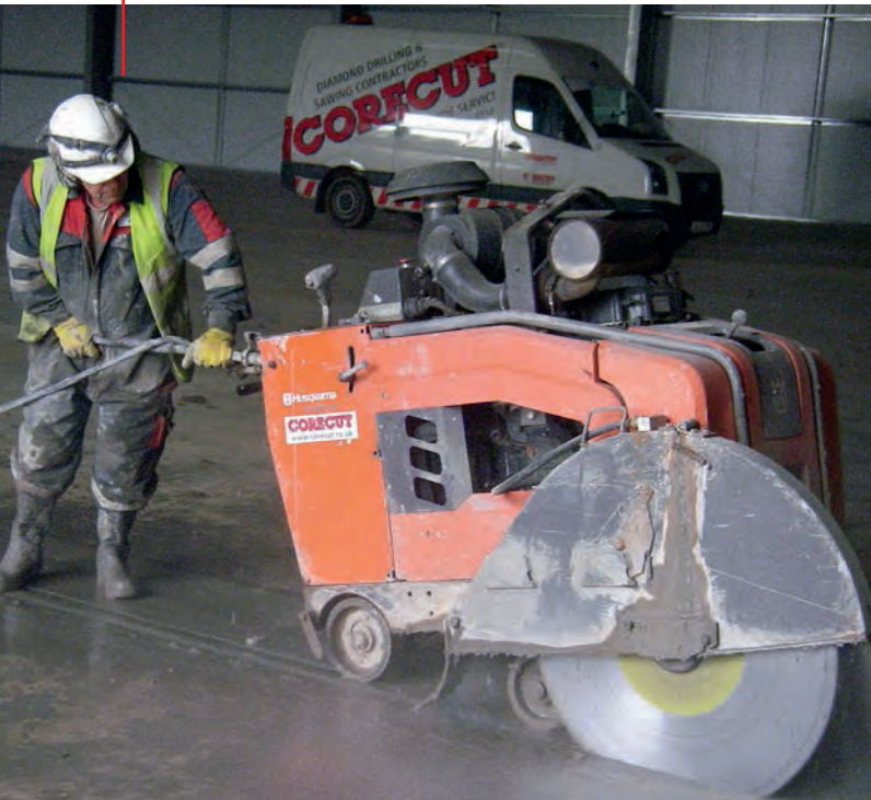
Floor Sawing to bonded warehouse floor
