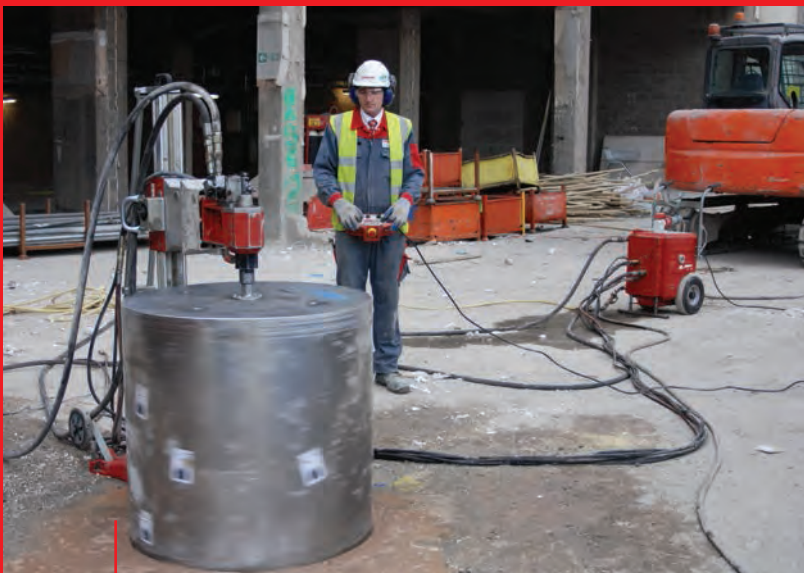
Large diameter drilling
