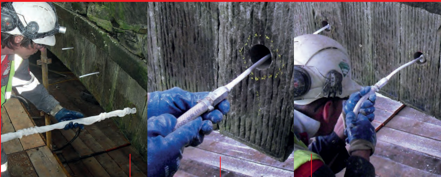
Cintec Anchor Installation
