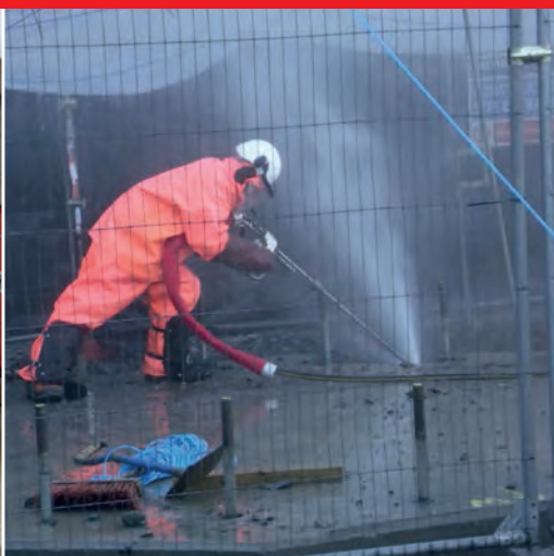
Handlancing to remove bolts
