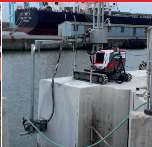
Robojetting provides solutions for difficult to access areas
