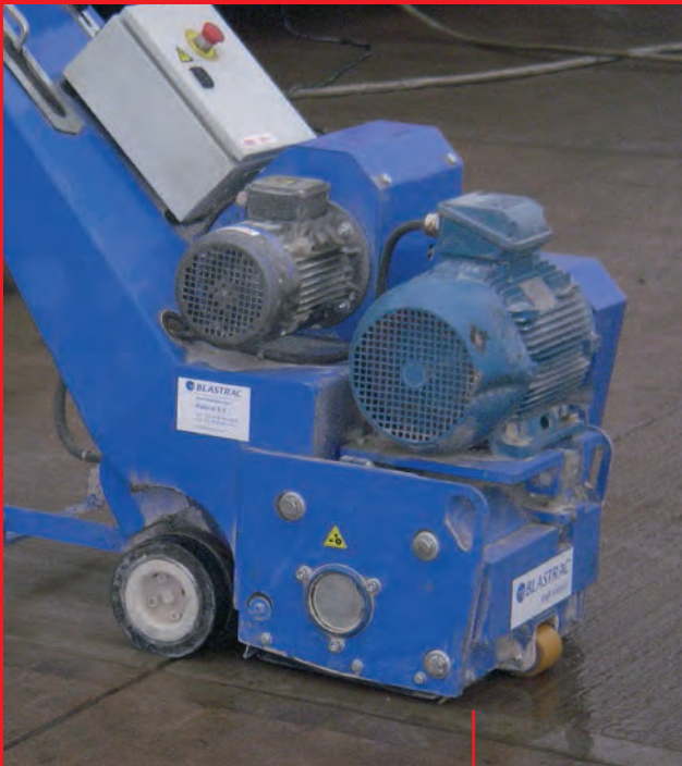
Grooving to provide texture to concrete car park
