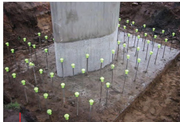
Installation of Starter Bars
