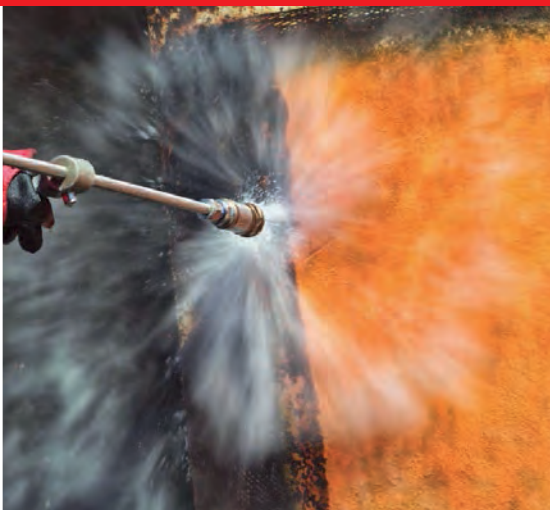
UHP Removal of Paint from Steel
