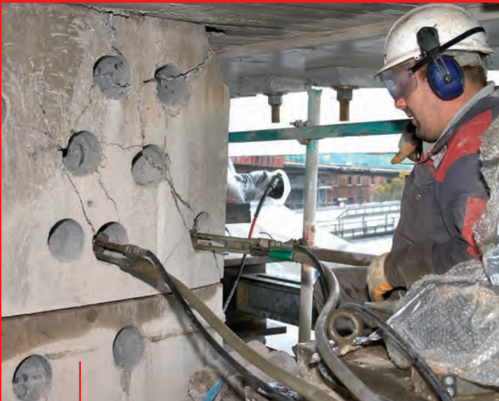
Removal of Bridge Columns
