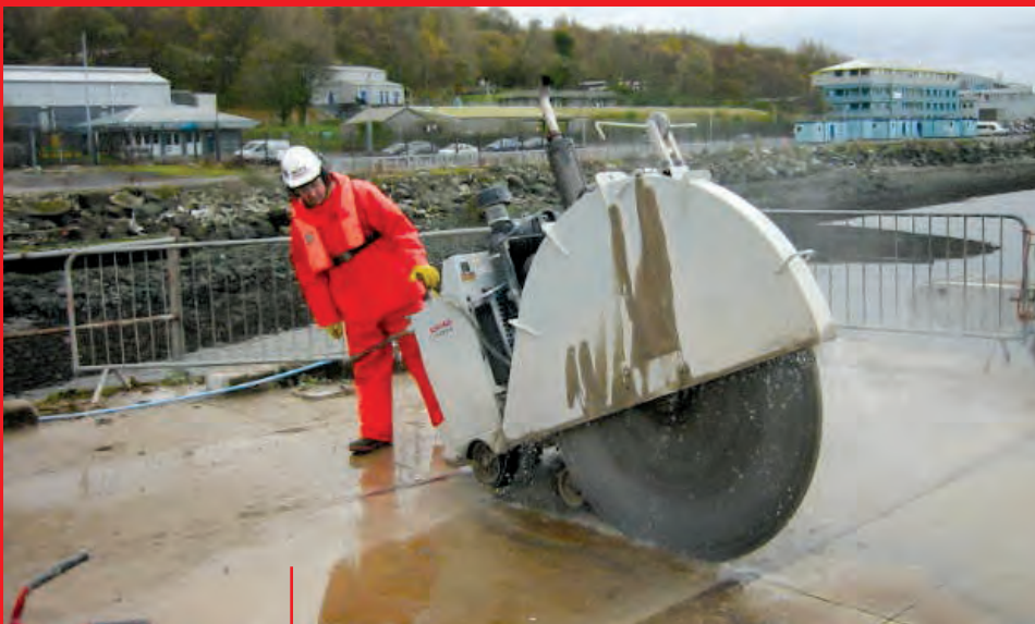
Cutting to 700mm depth
