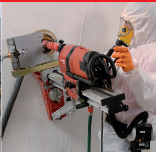
Dry Drilling with Full Dust Control
