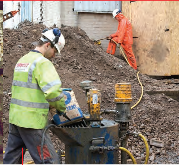
Grouting of Wall Cavity to Stabilise Structure
