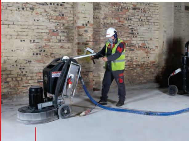
Concrete Polishing
