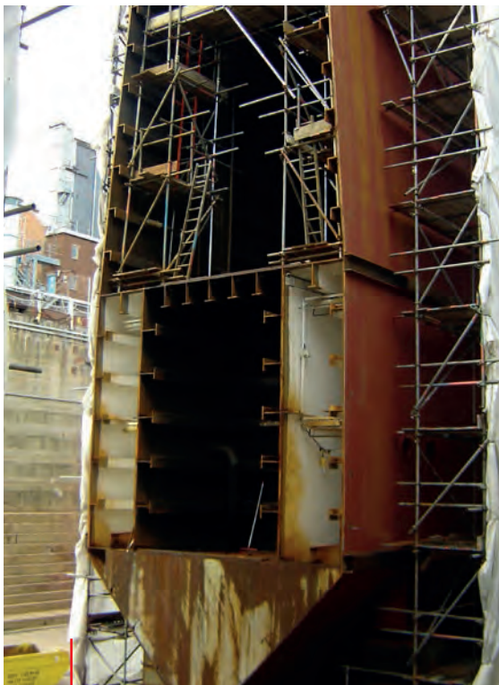
Wire Sawing Steel Caisson
