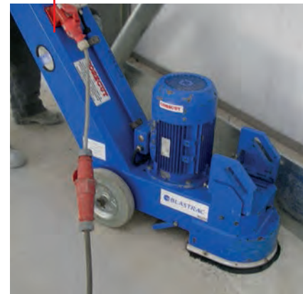
Concrete Grinding
