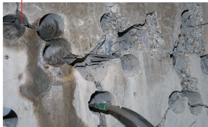
Controlled Demolition of Heavily Reinforced Concrete
