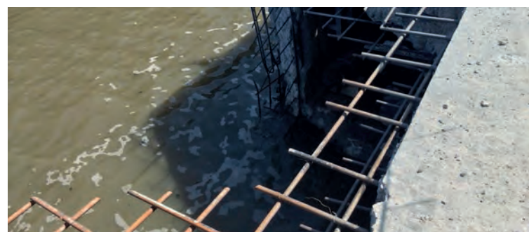
Hydrodemolition in Tidal Areas
