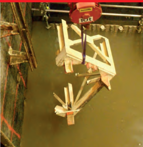
Removal by Remote Underwater cutting of steel framework
