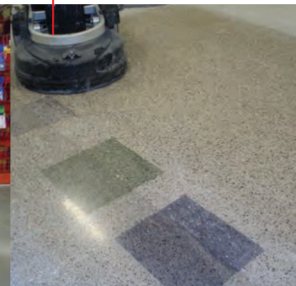
Stained Concrete Polishing
