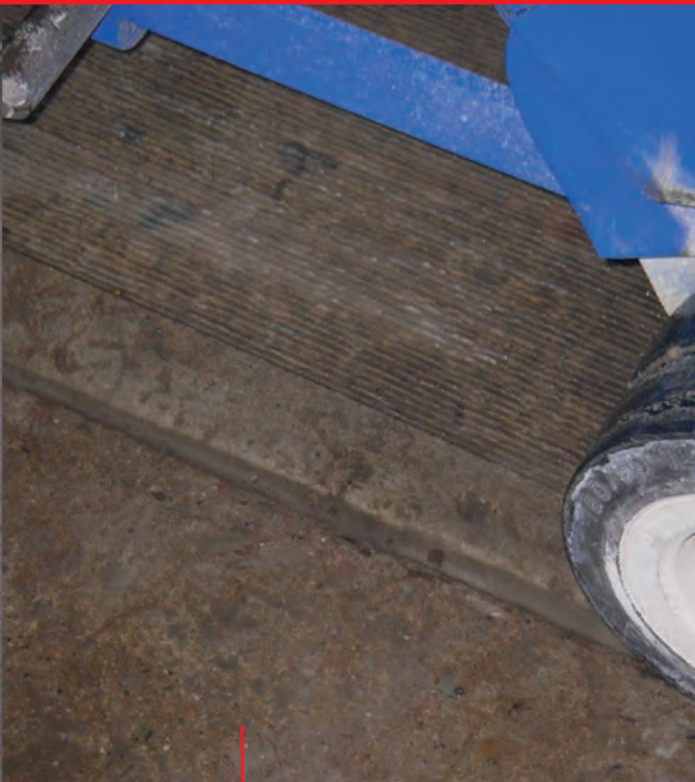
Grooving to provide texture to concrete car park
