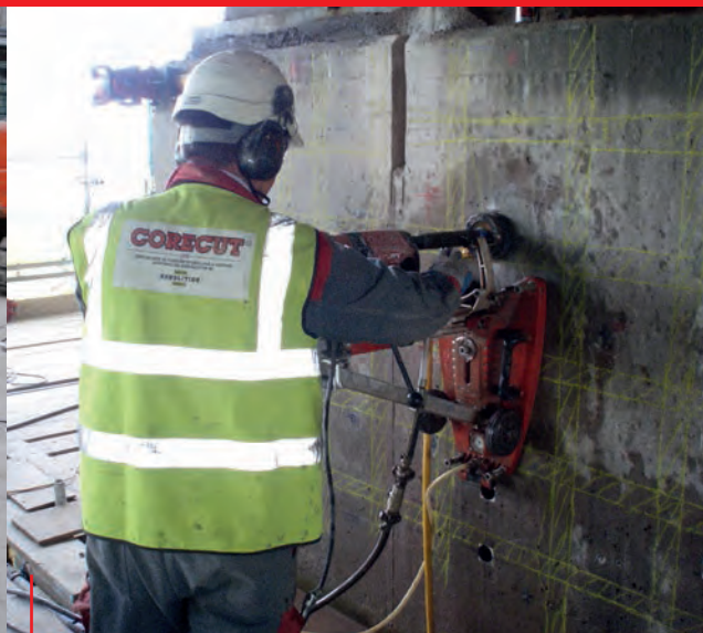
Diamond Drilling on the Forth Road Bridge
