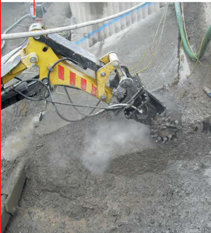
Drum Cutter profiling concrete
