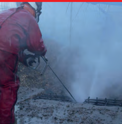
Precision Removal of Concrete by Hand Lancing
