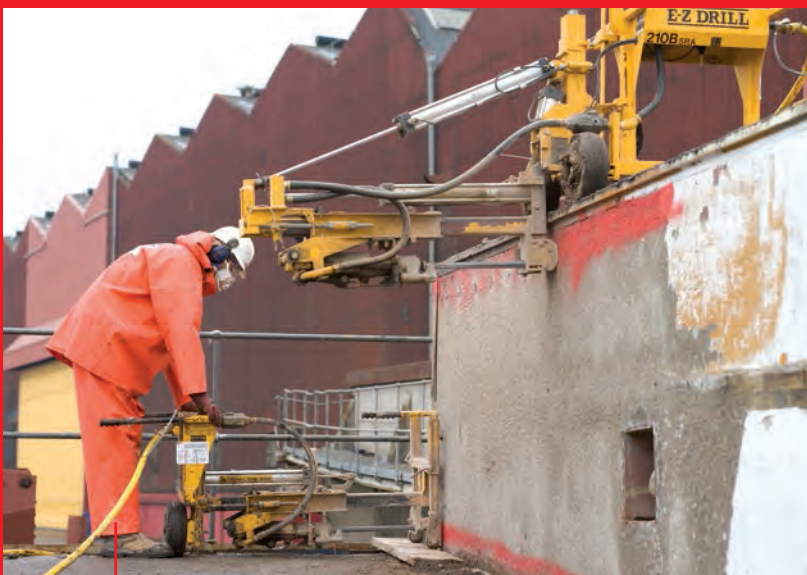
Rotary Percussive Drilling
