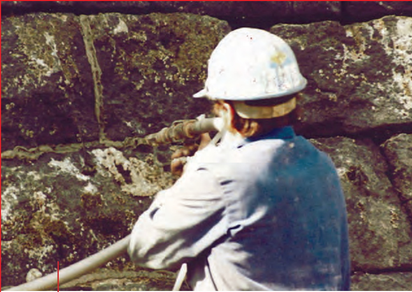
Pressure Pointing of Sea Wall
