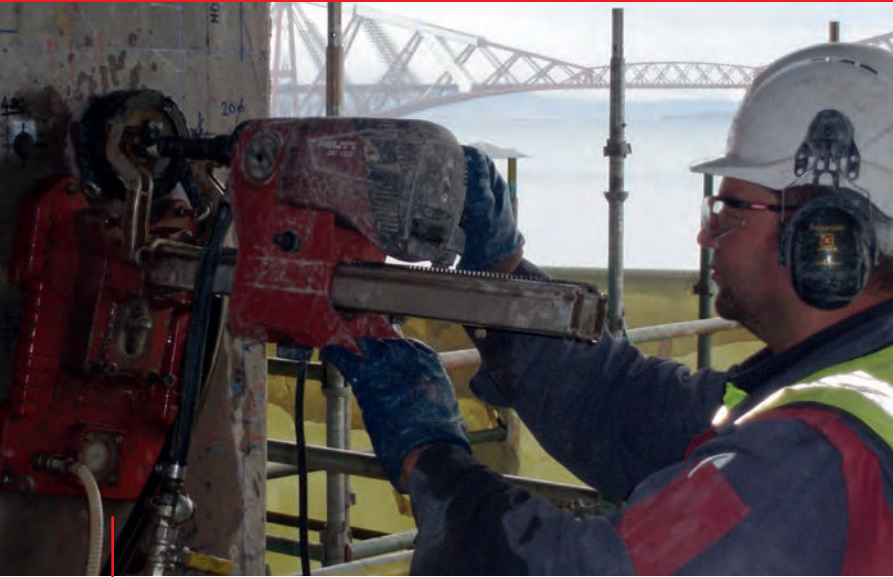
Diamond Drilling on the Forth Road Bridge
