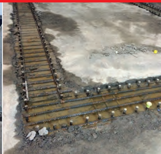
Precision removal of concrete
