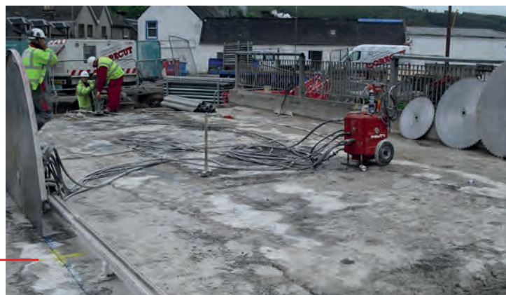
Cutting to Depths of 1000mm
