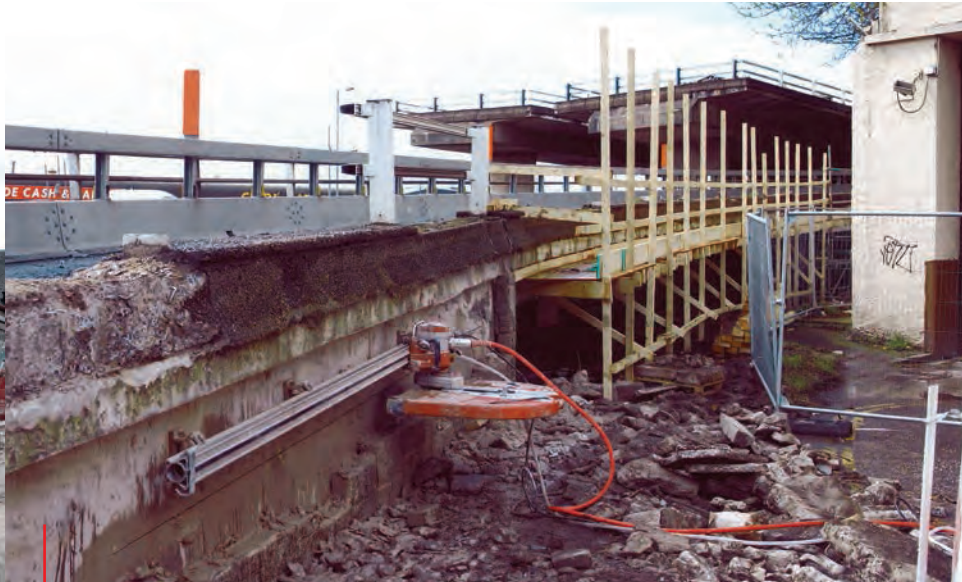
Pre-Cutting prior to Demolition
